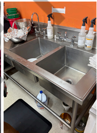
Sink at NW Corner
