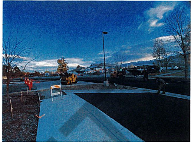
Road Paving and Sidewalks
