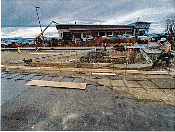
Gutter and Curb Work
